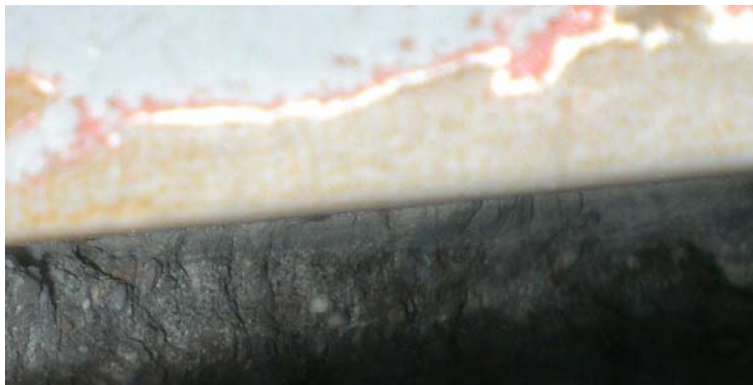
Figure 30 – Weak mortar grout caused by separation of the mortar, [9].
