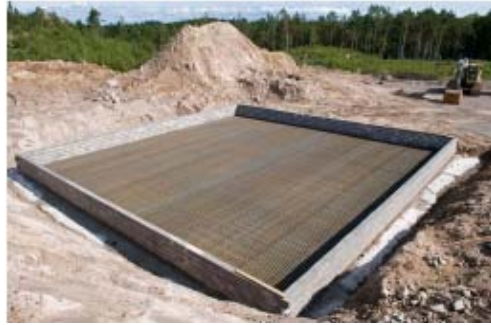
2- Bottom reinforcement
