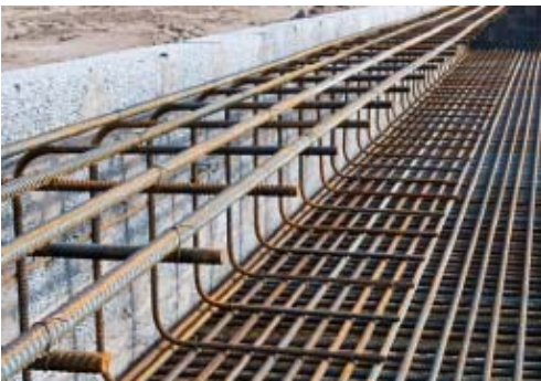
3- Bottom and edge reinforcement
