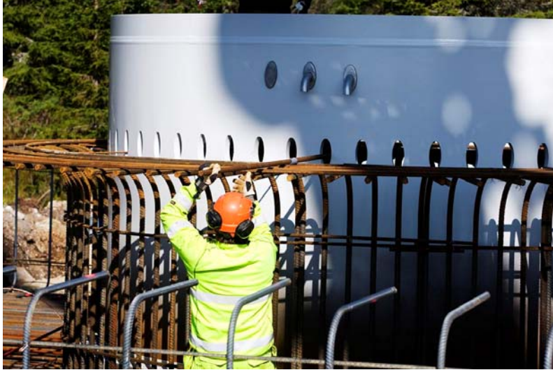
Figure 14 – Insert ring with holes through which the reinforcement bars pass.
