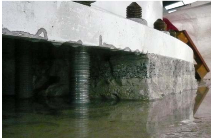
Figure 32 – Two different mortar grouts are used, [9].
