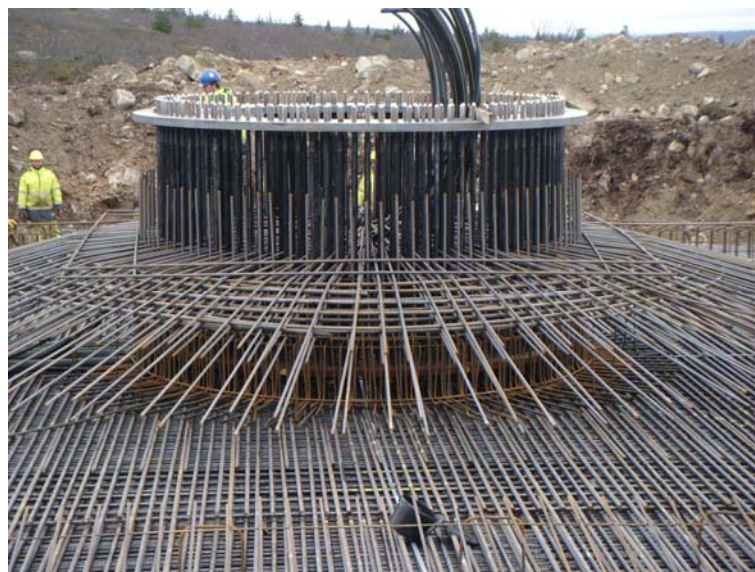
Figure 21 – Flange on the top of the pedestal before casting.
