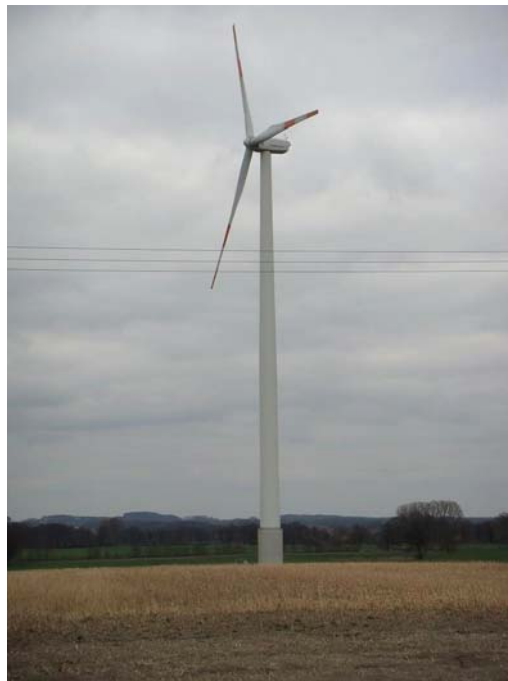
Figure 2 – Tubular steel tower on reinforced concrete pedestal.
