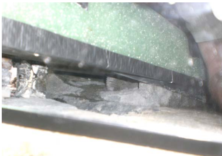
Figure 31 – Inclusion of air voids inside the mortar grout under the flange, [9].
