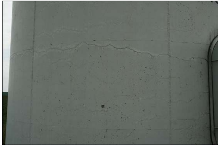
Figure 33 - Cracks in the reinforced door area, [15].
