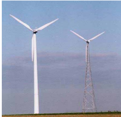
Figure 4 - A tubular and a lattice steel tower side by side.
