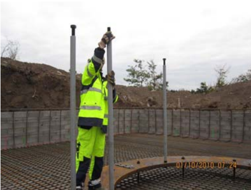
5- Stud bolts and bottom ring
