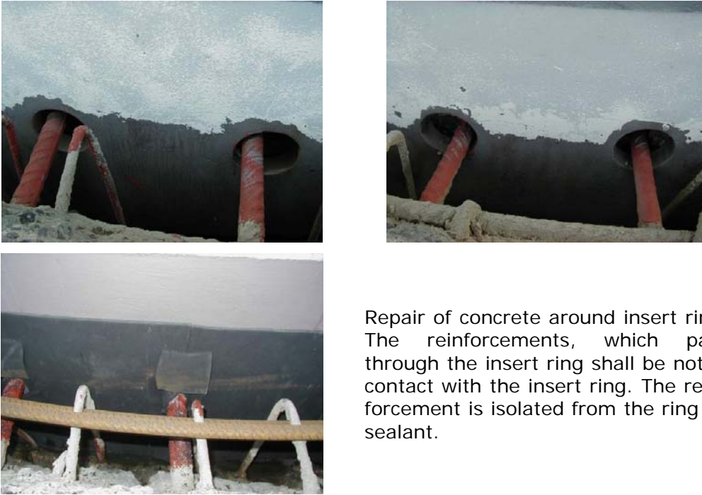
Figure 16 – Repair of concrete around insert ring, [9].
