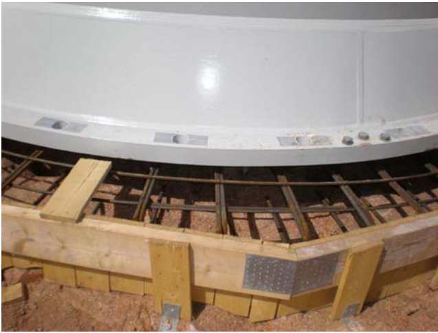
Figure 2 – Insert rings are also used for foundations on the bedrock.
