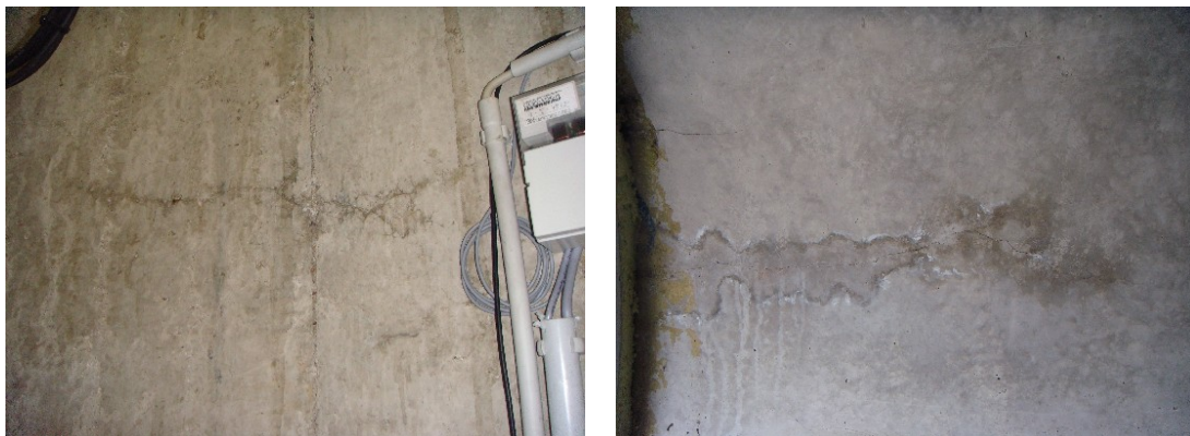
Figure 34 – Cracks on the concrete pedestal inside the structure, photo Hasanzadeh 2011.
