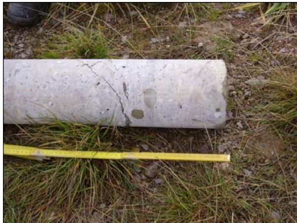
Figure 42 - Crack approximately 30 cm from the bottom of the foundation, [15].
